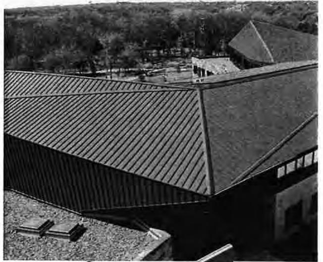
*The Berridge Cee-Lock Panel is an architectural metal standing seam panel that incorporates an integral snap-lock seam and an optional patented vinyl weatherseal.*
